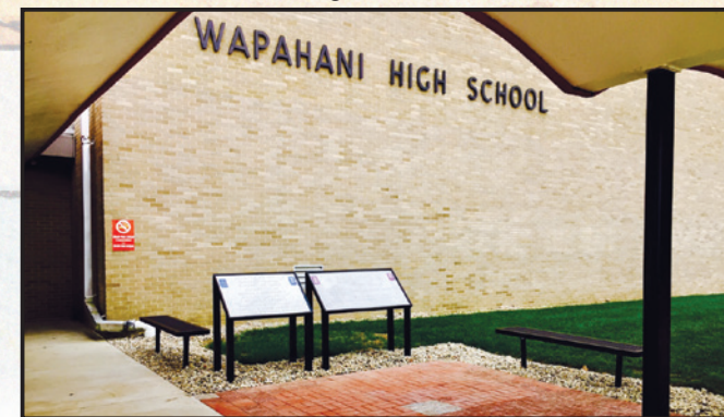
Highlighted above: 10.6' x 10.6' Walkway installed in NE corner of grassy area, West of the West Front Entrance of Wapahani High School.
